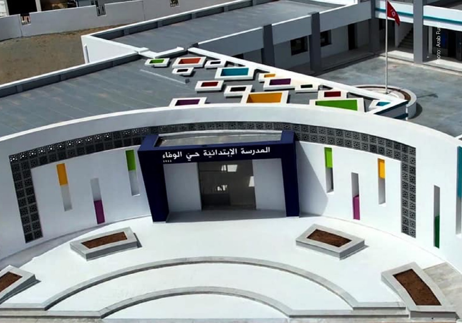
Al-Wafaa Primary School located in Nabeul, Tunisia
