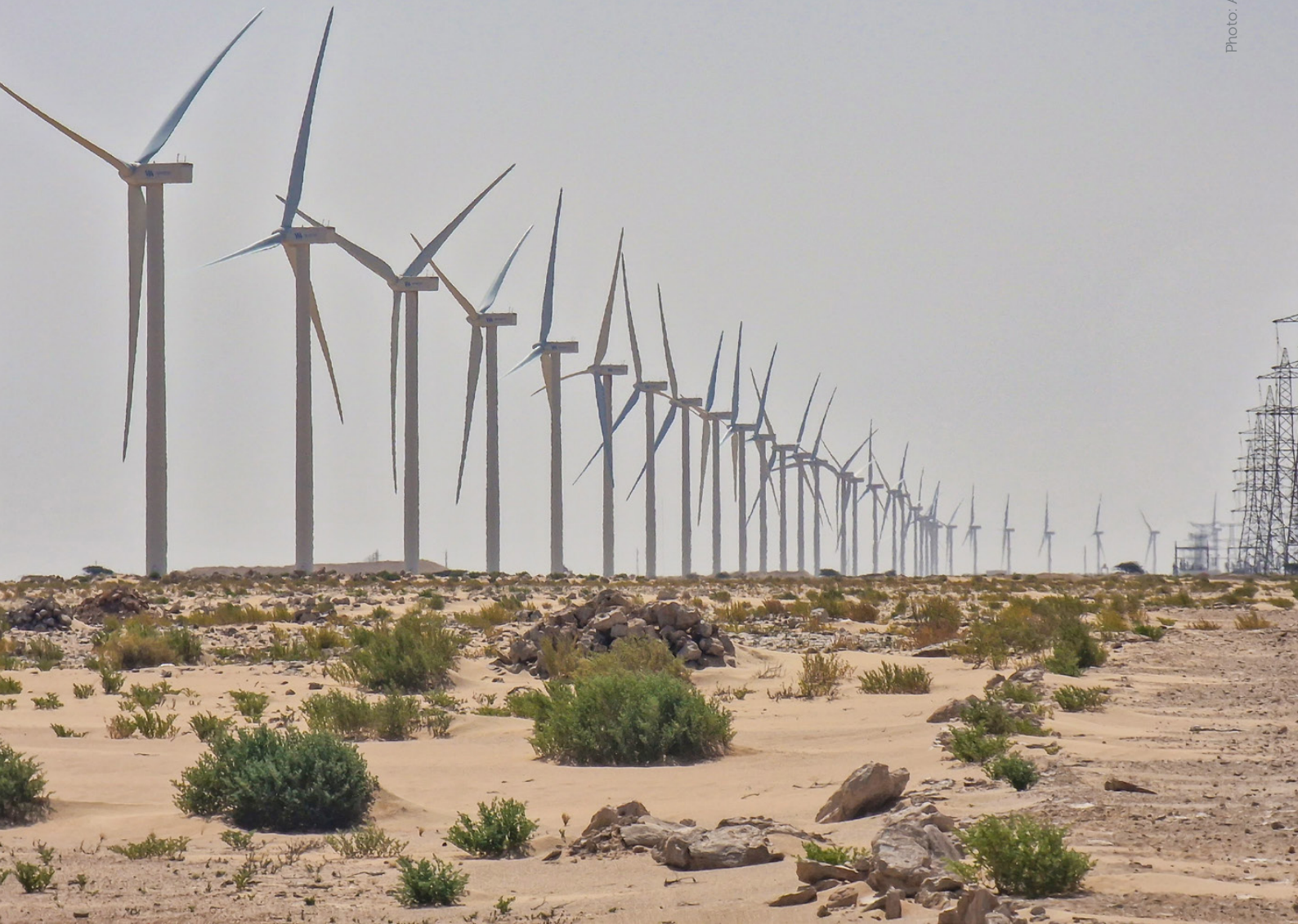
The Boulenouar Wind Power Plant Project in Mauritania
